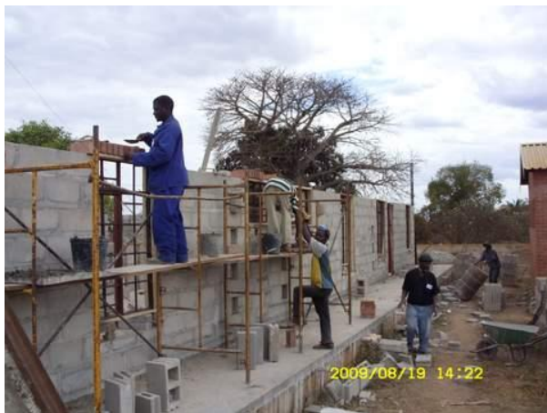
Erecting the rear wall of the building
