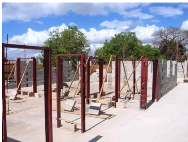
The future surgical block awaits the block layers
