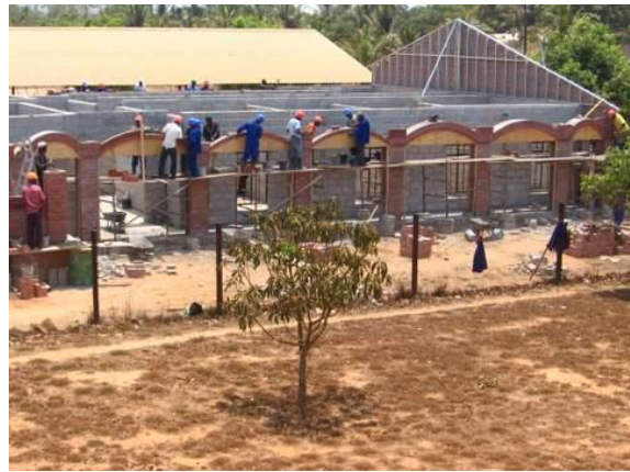
Workers build the arches on the clinic wing
