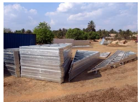
190 roof half-trusses await placement
