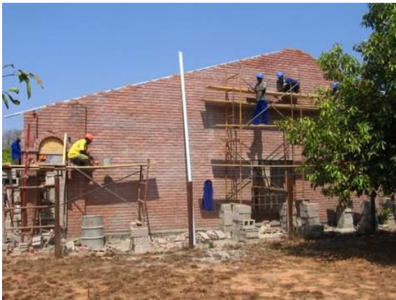
The east wall nears completion
