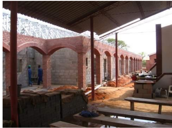
The rear arches completed
