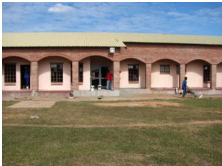
The outside of the hospital, painted and with security lights in place
